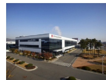
[LGES Ochang Battery Factory - GS E&C]
