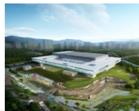
[Suwon Convention Center - Hanwha Construction]
